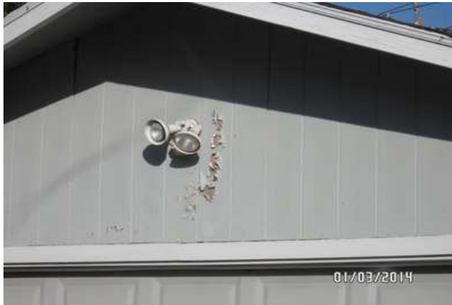
Minor Damage Paint peeling
