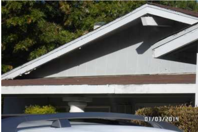
Paint Peeling at fascia and no gutter.
